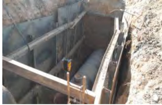
Trench Less Work at Railway crossing near IOCL, Noonmati in progress
