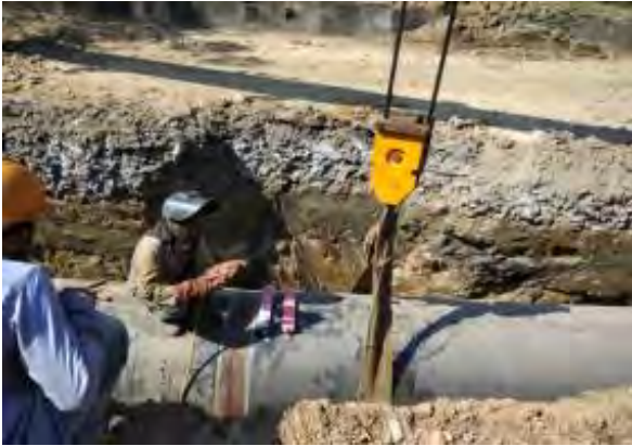
Joining of pipe by welding at VIP road
