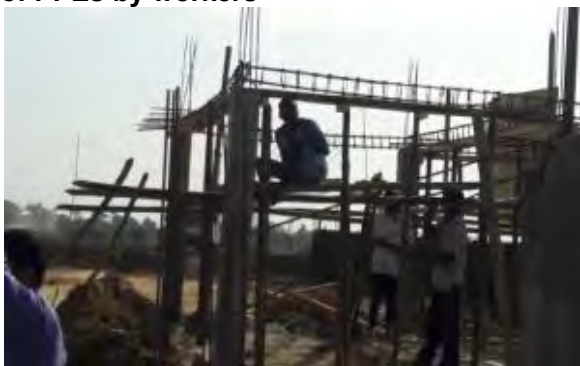
Security Guard room under construction
