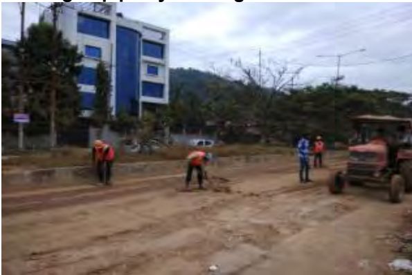
Cleaning of the road after filling of trench
