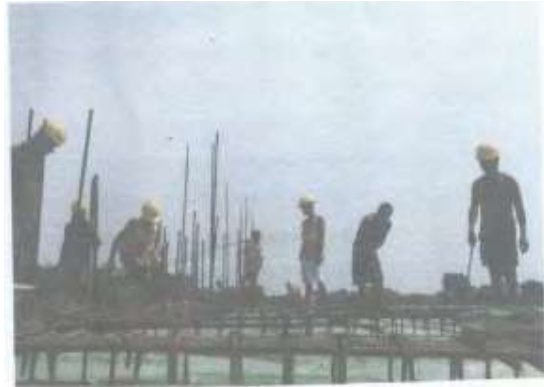
Use of PPEs during construction – noted
