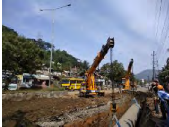
Lowering of pipe for laying
