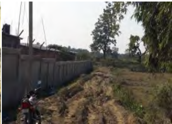
Compound wall of landfill constructed
