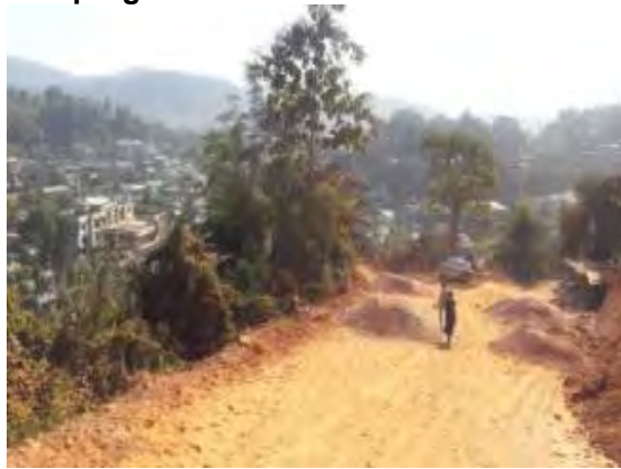
Approach road under construction
