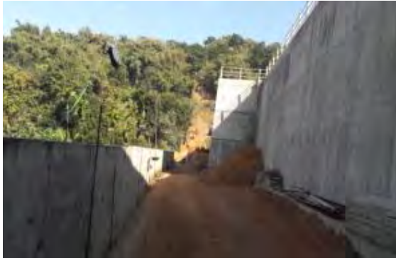
Final stage reservoir construction work continued at Gopalnagar
