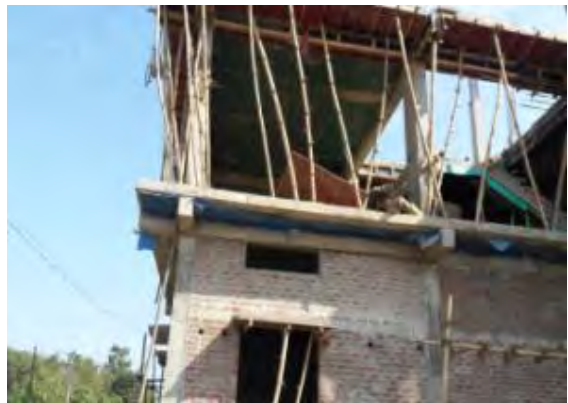
Administrative building under construction at landfill site
