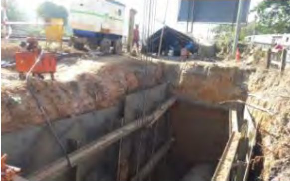
Shoring is noted for pipe laying. Area closed by caution tape
