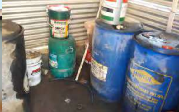
Storage of fuel noted within close room. No use of oil tray below the fuel drum. Land contaminated.
