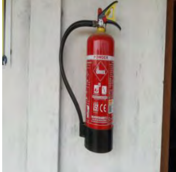
Fire extinguisher noted at office and near the fuel store
