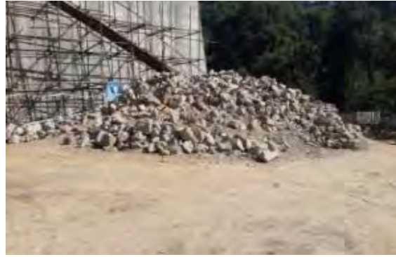
Stone/ boulders after utilization needs to be removed from work site
