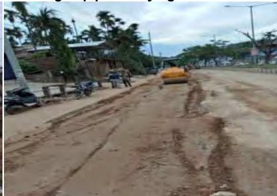
Temporary road restoration at VIP road
