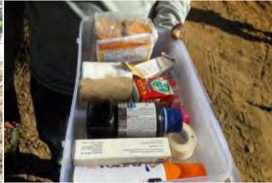
First aid box noted at work site
