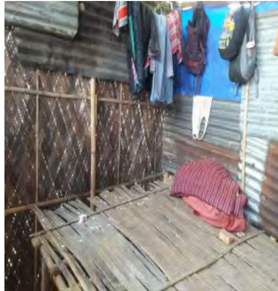
Labour camp. No proper bed
